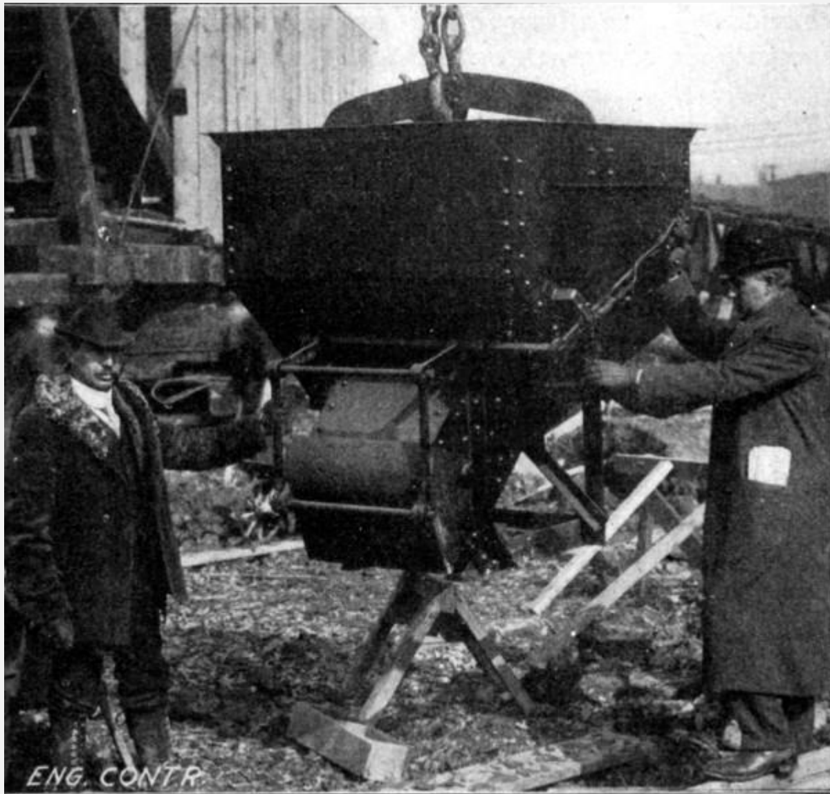
g. 222.—Special Concrete Bucket for Large Warehouse Building.
