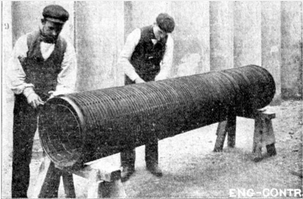
g. 271.—Applying External Reinforcement to Bordenave Pipe.
