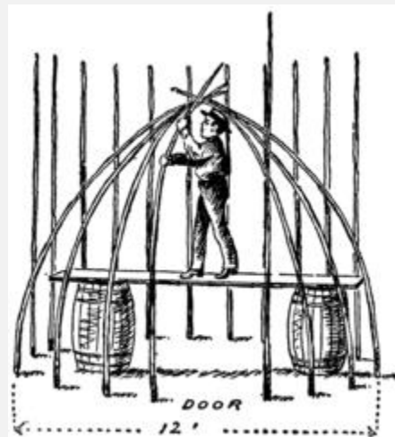
Fig. 131. Making the Frame of the Straw Hut.
