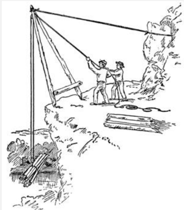
Fig. 137. The Derrick in Use.
