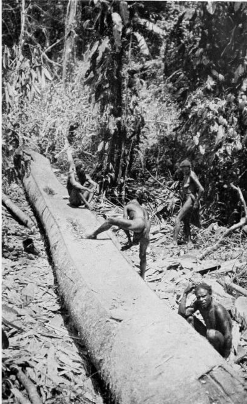
CANOE-MAKING: ROUGHLY SHAPING THE FELLED TREE.
