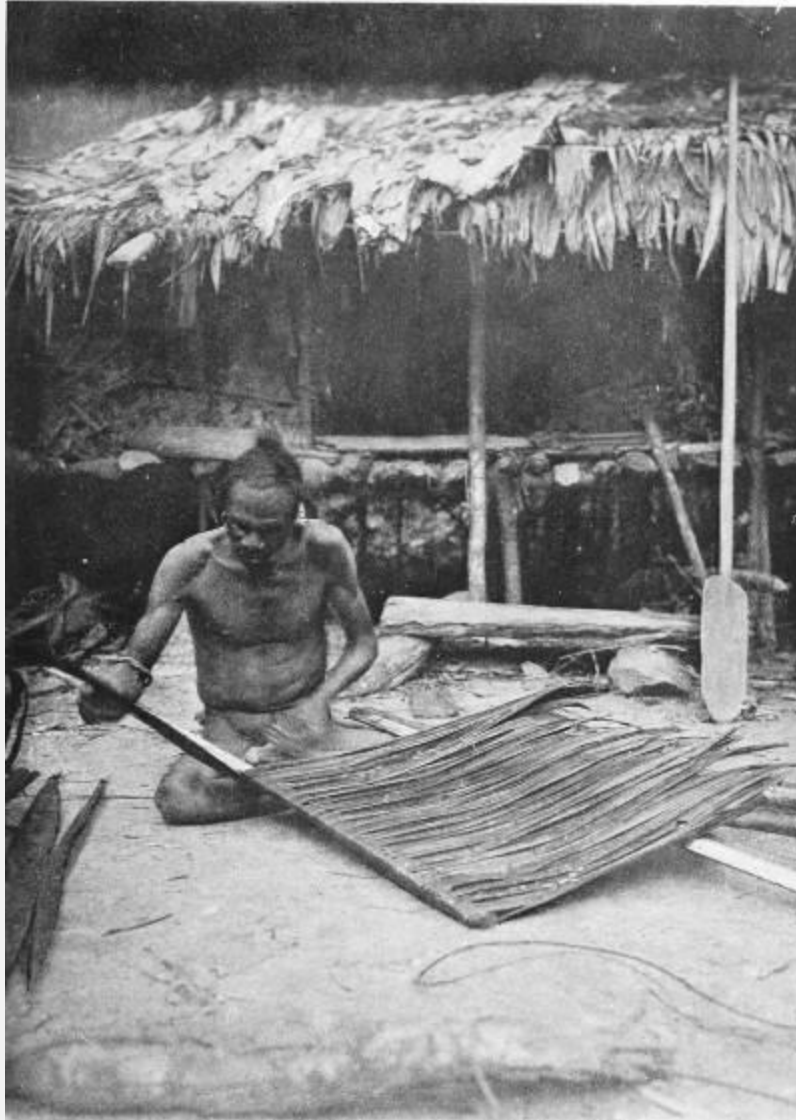
MAKING “ATAP” FOR ROOFING.
