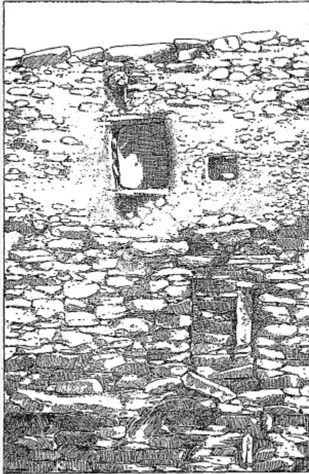
FIG. 92. Sealed openings in Tusayan.
